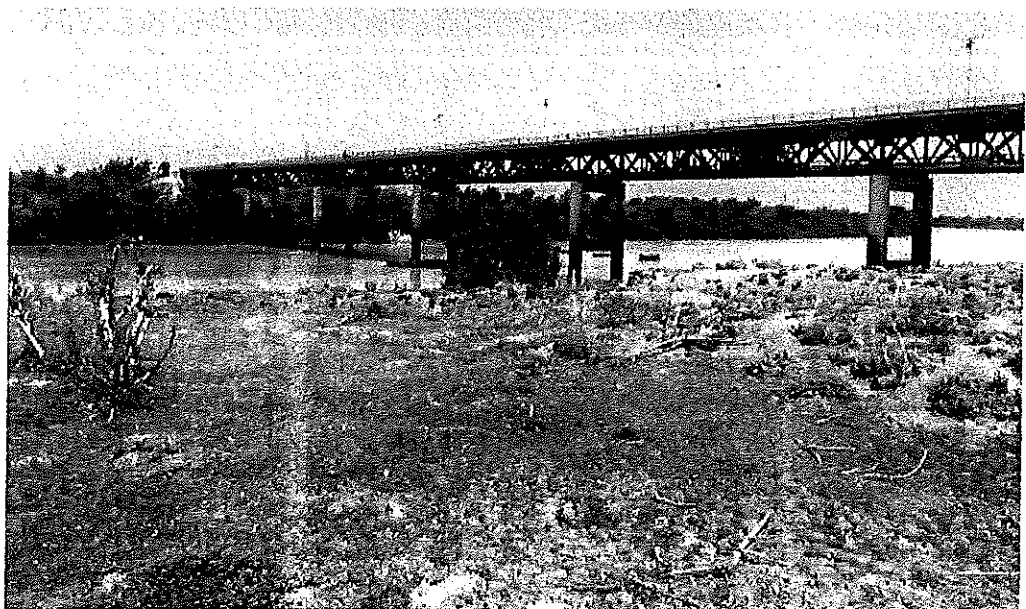
Figure 12. Yapei Bridge. Elevation view. Spans over riverbed.
