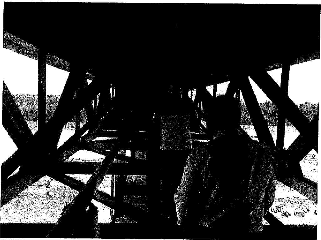
Figure 16. Yapei Bridge. Visual inspection through a walkway on the steel truss.
