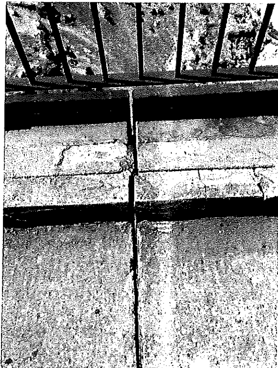
Figure 24. Yapei Bridge. Detail of Intermediate joint between lab segments.
