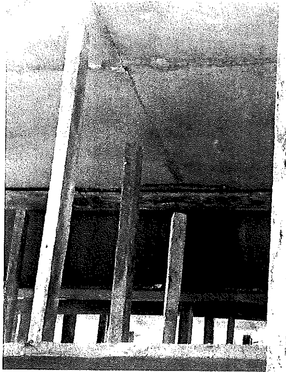
Figure 19. Yapei Bridge. Remaining support scaffolding wood elements used in recent intervention.
