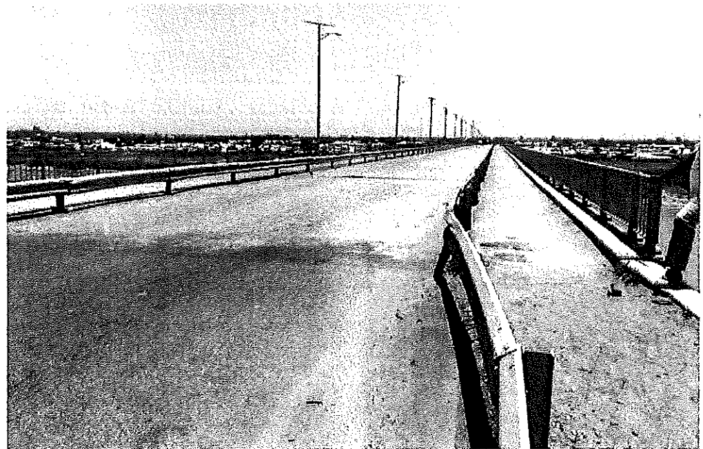
Figure 10. Bulpe Bridge. Bridge deck platform and sidewalks.
