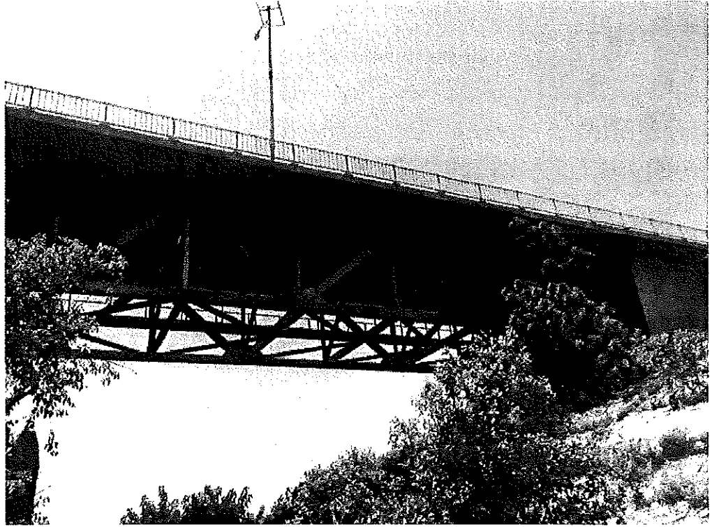
Figure 5. Bulpes Bridge. General view of side span.
