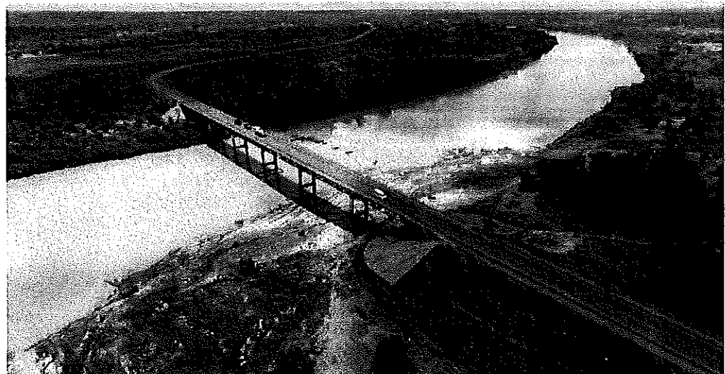
Figure 2. Aerial view of Yapei Bridge over White Volta, towards west.
