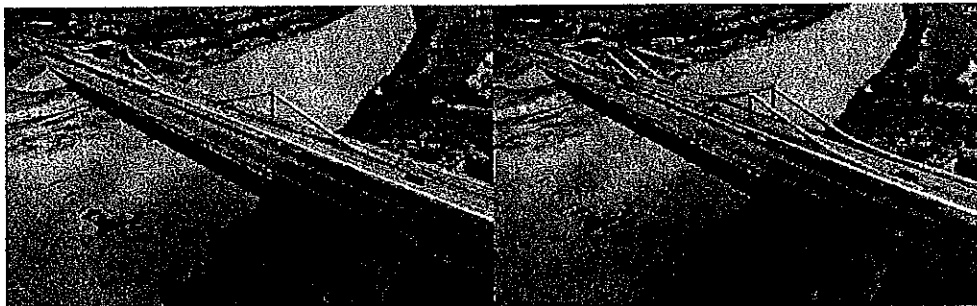
Figure 10 –Proposals with one plane of stay-cables or with two planes of stay-cables
