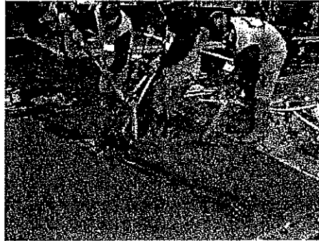
Figure 27- Concrete Leveling
